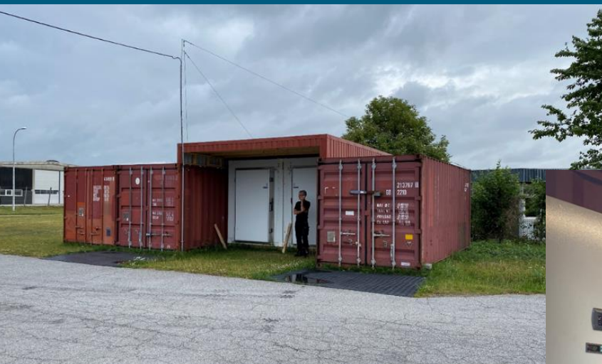
Provision chambers & Engine room
